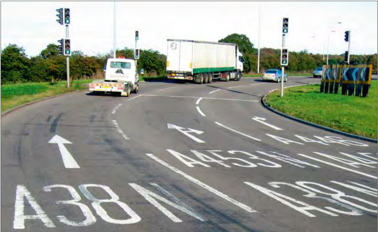
Figure 4.13 Lane markings – arrows and destinations on circulatory carriageway
