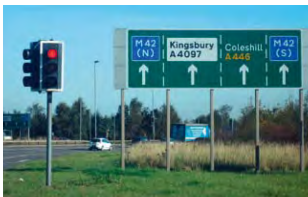
Figure 4.14 Lane destination signs
