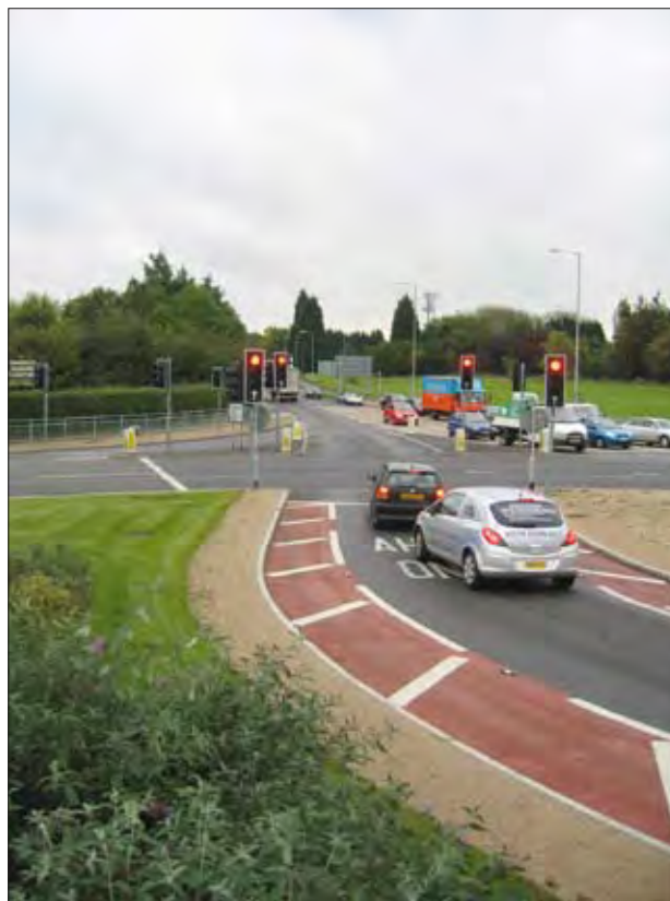
Figure A.2 Bardills roundabout showing cut-through (looking towards arm A, Stapleford Road).
