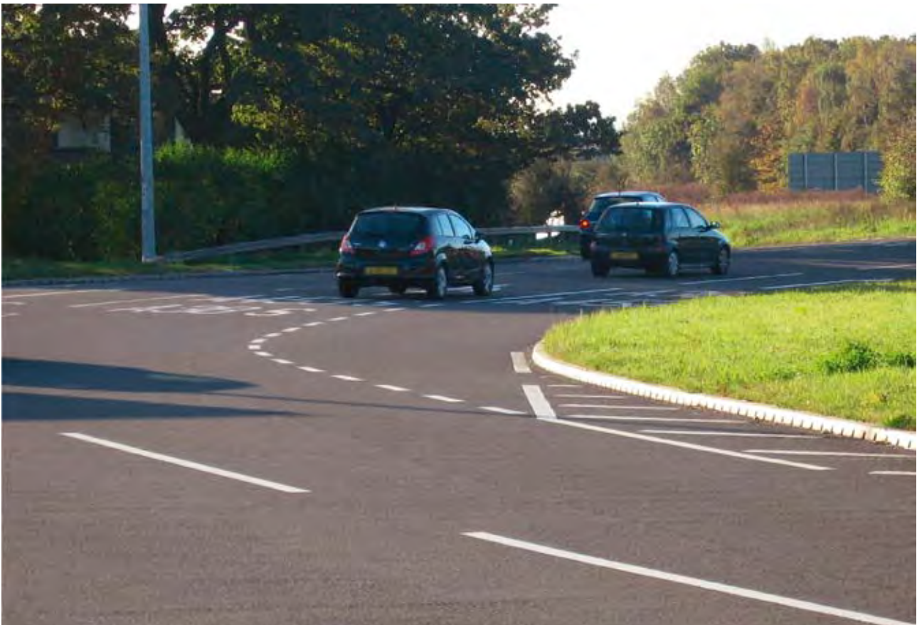
Figure 4.11 Spiral markings and hatching
